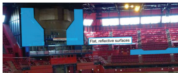
Figure 2. Reflecting surfaces causing adverse echoes
