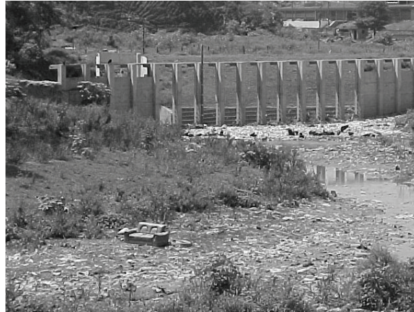
Figure 3 – Solid waste in a detention reservoir (Orsini, 2001)
