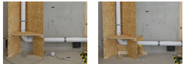
Figure 20: Bend at bottom without (left) and with additional 25 mm OSB shielding (right). Note: Care was taken to have no contact between OSB plates and pipe or reception plate.
