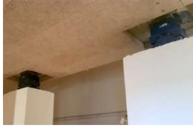
Figure 17: Example of the elastic supports of the chambers of the acoustic laboratory.
