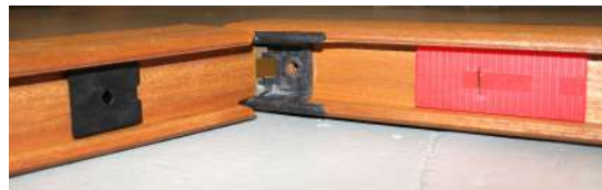
Figure 2: Connection between the leaf and the sash of the casements.
