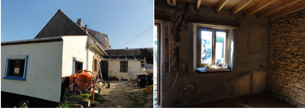
Figure 4: Housing in hand to renovate
