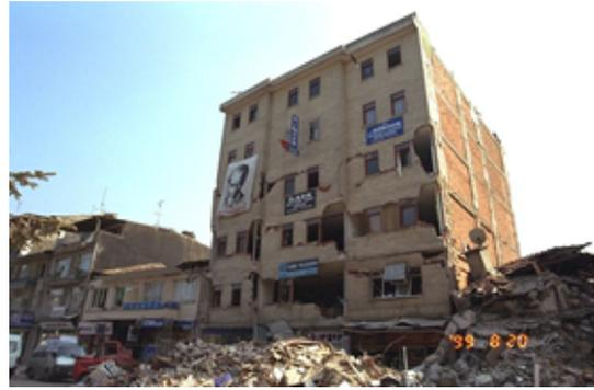
(b) Pounding damage to the reinforced concrete frame and masonry infill building observed during the Mw 7.4, Izmit earthquake, Turkey, 1999[6]
