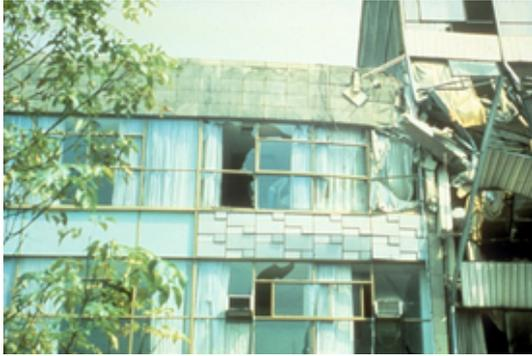
(a) Intermediate floor collapse (mid-story) of Hotel de Carlo in Mexico City, probably caused by pounding against the shorter building to the left; photograph taken after the Mw 8.1 Mexico earthquake[5]
