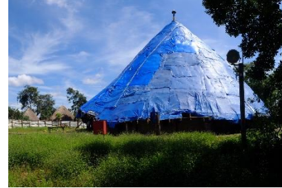
The ceiling must be protected from rain with a tarpaulin during the work
