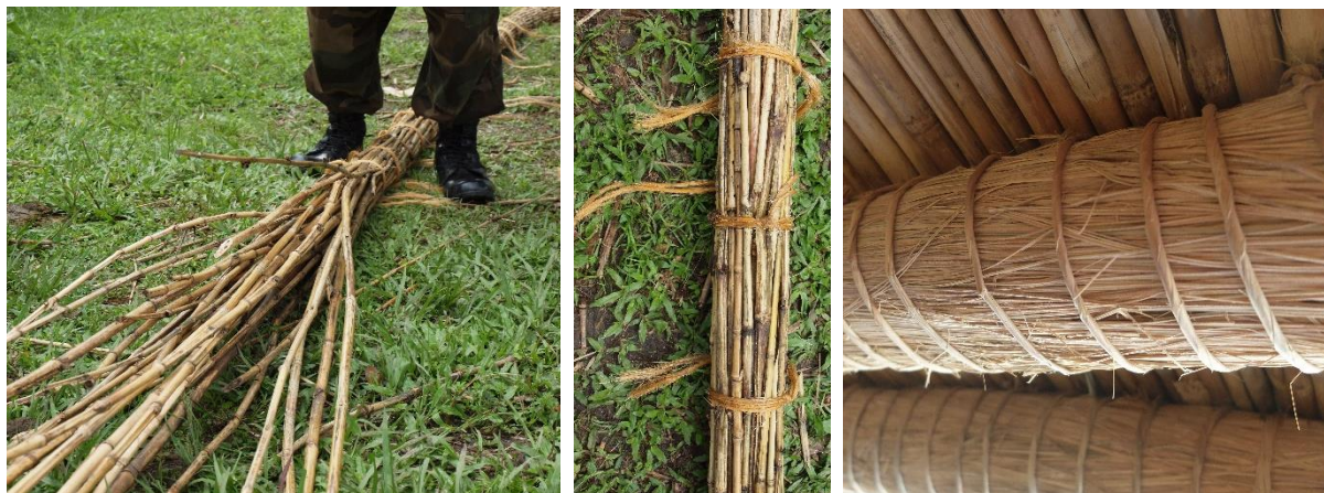
Tying the reeds with sisal rope to prefabricate rings
