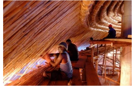
Inserting the reeds by force from below
