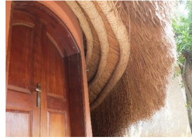
Example of ceiling edge neatly cut
