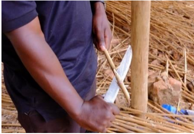
Sharpening the reeds end
