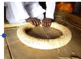
Prefabricating the rings.
