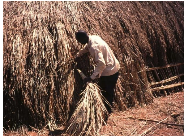
Insertion of new bundles at the base of BujjaBukula, Kasubi
