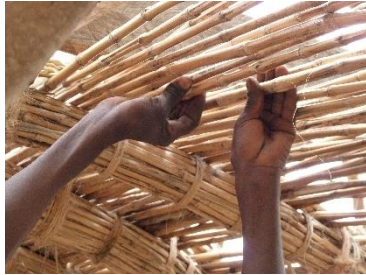
Inserting the reeds by force from below
