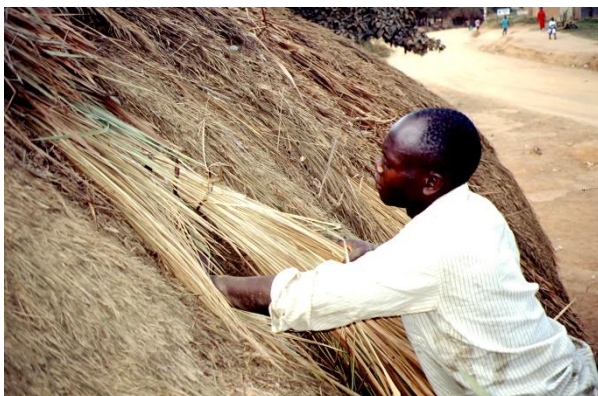
Inserting new bundles in a gully after removing decayed grass
