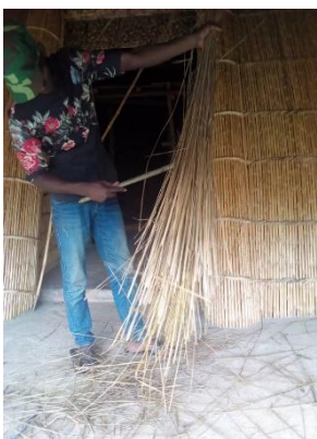
Combing a bundle with a stick to remove unwanted elements and tying the bundle in a conical shape with a sisal rope 4 photos by Brian Kalema
