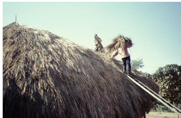
Bringing new spear grass bundles on the roof to fill gullies
