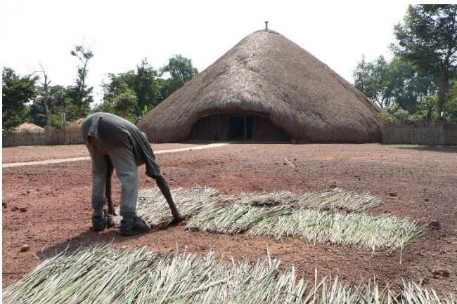
Laying spear grass on the ground for drying and removing unsuitable elements (other plants and broken stems)
