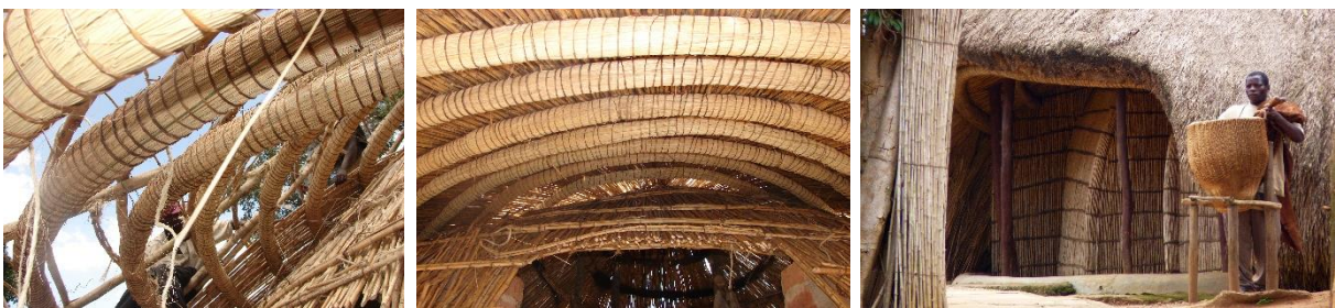
Details on the extra ceiling covering the entrance 2 photos by Remigious Kigongo
