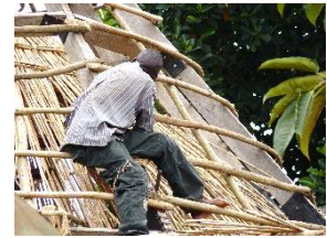
Workers sitting on the battens to work on the ceiling.
