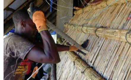
Adjusting the position of the reeds
