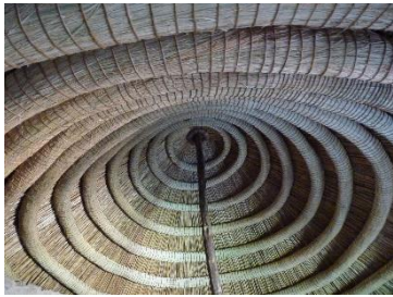
The rings are wrapped at the end with palm frond sticks and water grass
