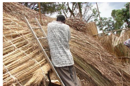
Tying thatch bundles to the battens 3 photos by Remigious Kigongo
