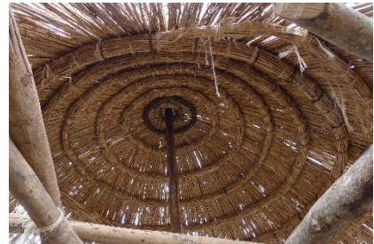
Upper part of the ceiling done
