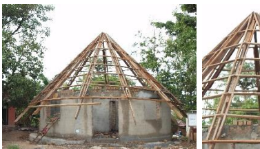
Timber skeleton, mixing 2x5" and 2x3" rafters, Kajjaga , Kasubi
