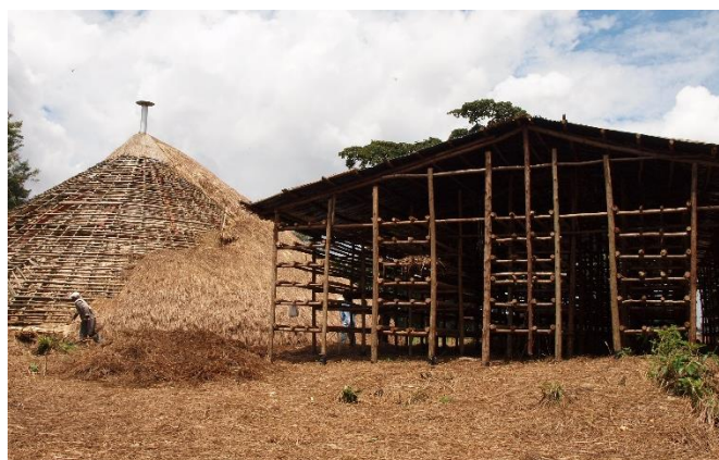
Shed for keeping spare dry grass at Wamala
