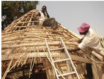
Team work: one pushes the reeds and the other adjusts the position photo Remigious Kigongo
