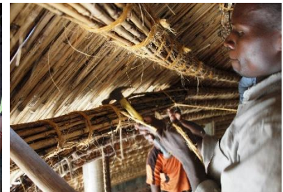
pulling a ring with a hammer
