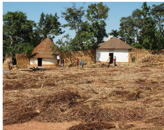
Laying spear grass on the ground for drying and removing unsuitable elements (other plants and broken stems)
