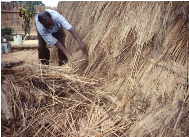
Removal of decayed thatch at Kasubi
