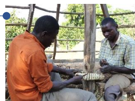
Manufacturing the first ring around the pole.
