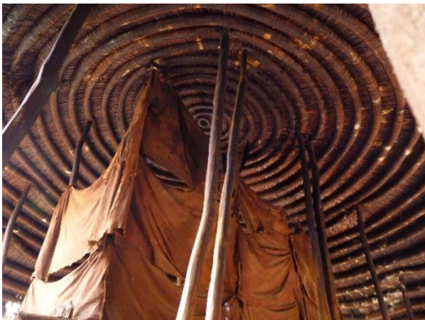
Rings protected by a layer of suit at Wamala tombs.
