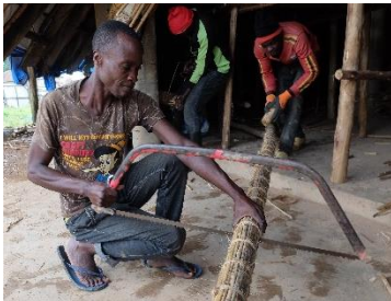
Cutting a prefabricated ring to the right size
