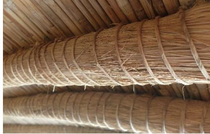
The rings are wrapped at the end with palm frond sticks and water grass
