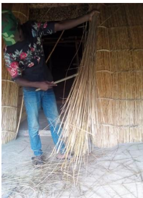
Combing a bundle with a stick to remove unwanted elements and tying the bundle in a conical shape with a sisal rope 4 photos by Brian Kalema
