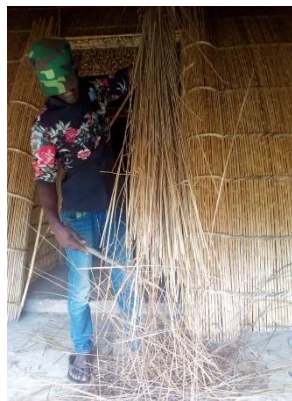
Combing a bundle with a stick to remove unwanted elements and tying the bundle in a conical shape with a sisal rope 4 photos by Brian Kalema
