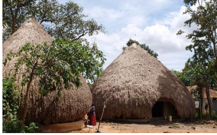
The thatch should not touch the ground
