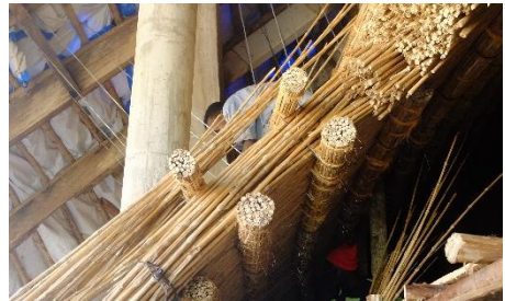
Section on the ceiling at the door level. Lower and upper rings are attached with binding wire
