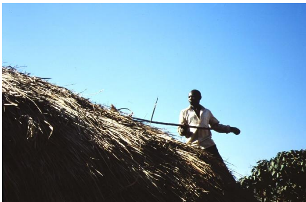
Cleaning and readjusting the thatch with a stick
