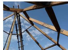
Timber skeleton, using 2x6" rafters, Balongo Abawenda house, Kasubi
