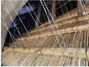
2 mm steel wires connecting the ceiling to the battens
