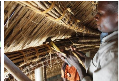
pulling a ring with a hammer
