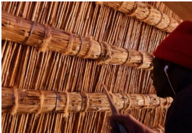
Adjusting the reeds position to avoid overlaps
