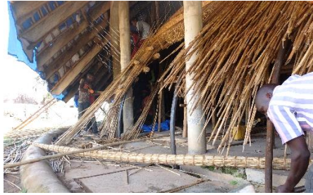
The reeds are not cut at the bottom until the work is finished
