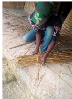
Combing a bundle with a stick to remove unwanted elements and tying the bundle in a conical shape with a sisal rope 4 photos by Brian Kalema
