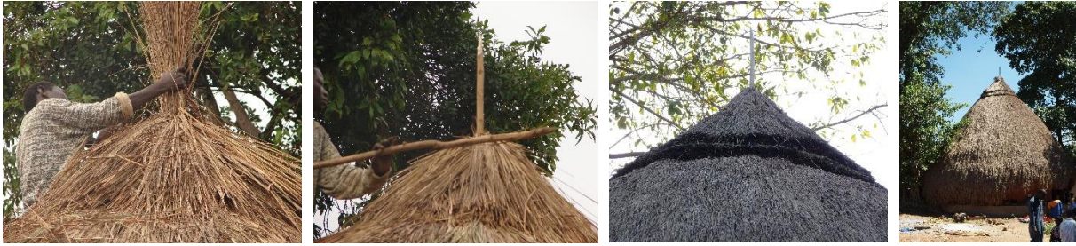
Examples of top finishes 2 photos on the left by Remigious Kigongo
