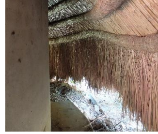
The thatch should not touch the ground
