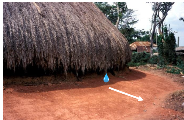
Drainage slopes made of compacted laterite
