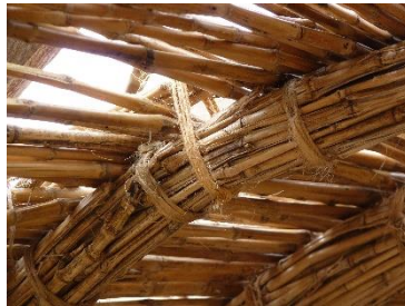
Lower and upper rings attached with a sisal rope
