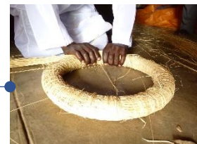
Prefabricating the rings.
