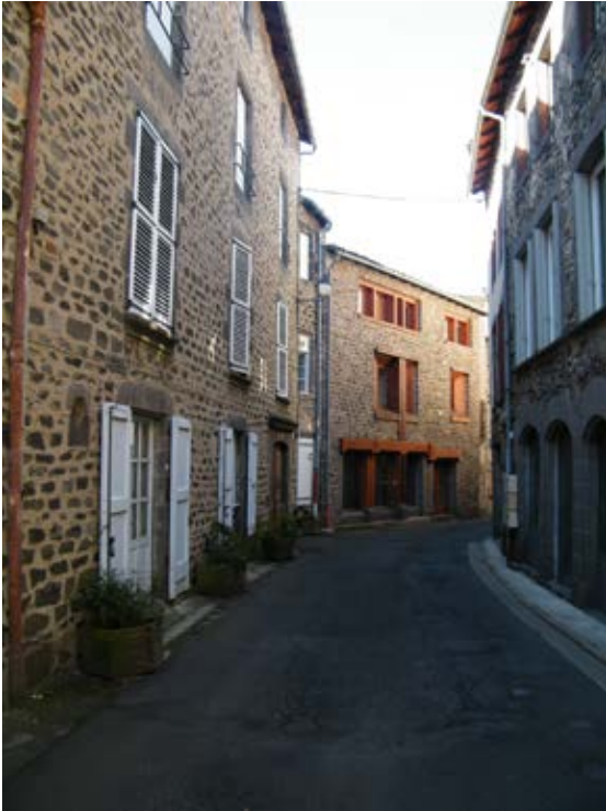
Works of facade : rehabilitation well advanced
