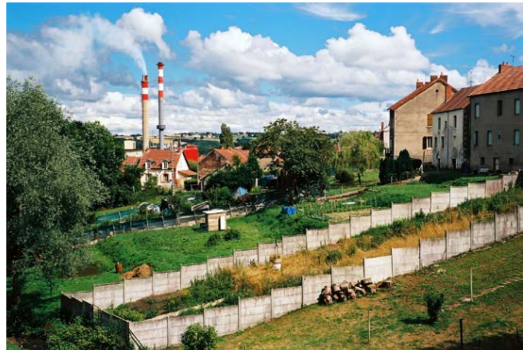
The industrial reconversion with the international company «Rockwool Insulation»
