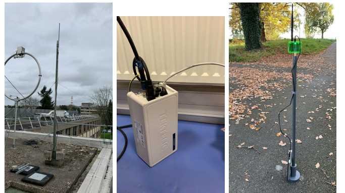
(a) Position of the gateway monopole antenna fixed on a roof. (b) The gateway component fixed to the antenna rod and connected to a cable. (c) The packaged Pycom device fixed on a battery at location 7.
