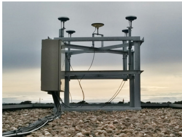
(A) Antenna platform.
