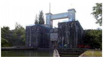
*Illustration 2: Downstream part of the lock with the lower gate and its mask-girders.*
