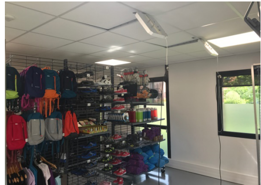
FIGURE 5. Two Laird antennae mounted overhead, above the shelves (case B).
