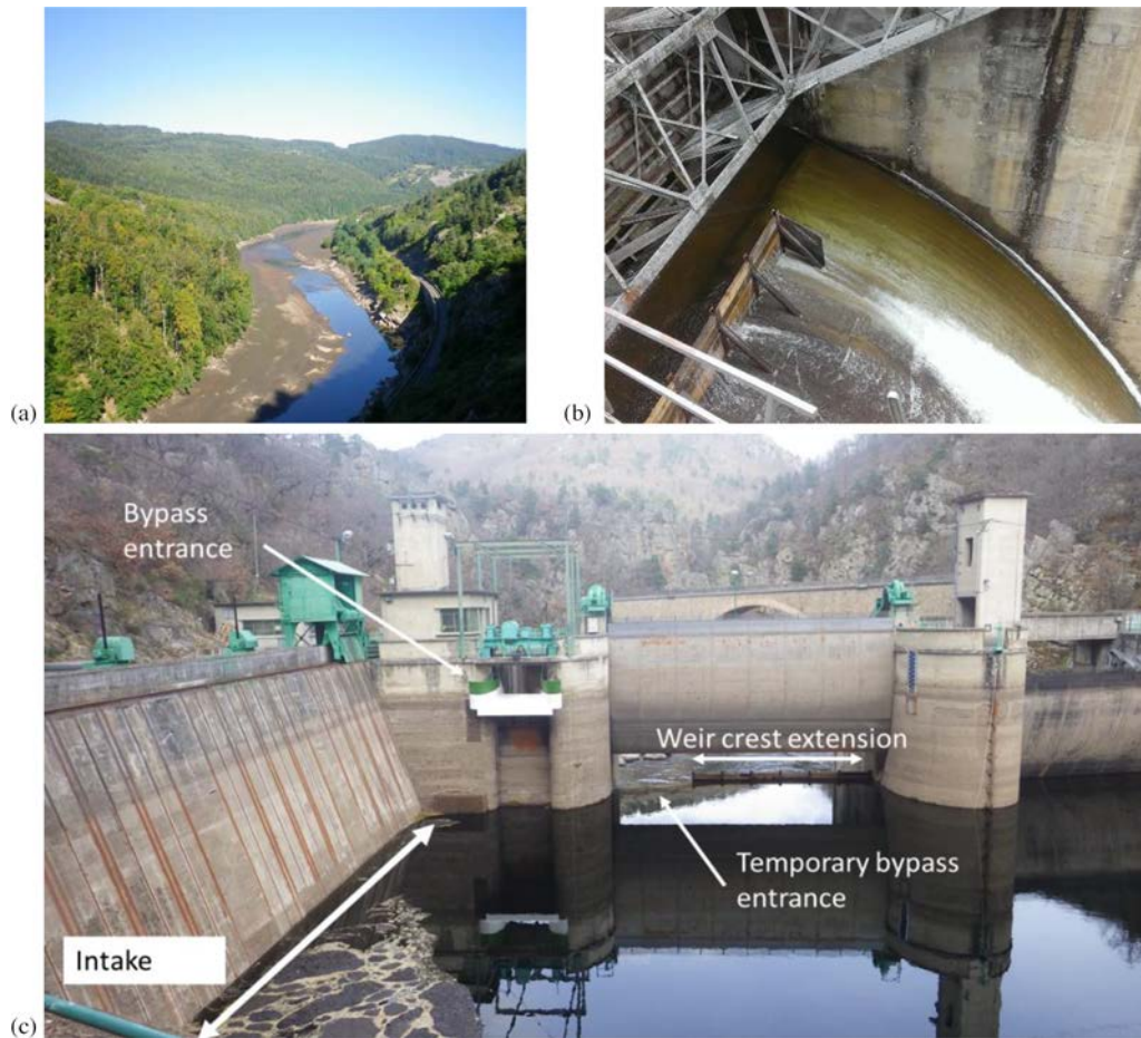
Fig. 3. Picture of upstream limit of the temporary Poutès reservoir (a). Top view of temporary bypass (b). Upstream view of intake, usual (non functional) and temporary bypass entrances (c).
