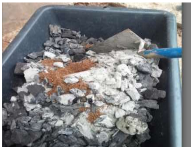
Figure 25 Dry mixing of different constituents of concrete
