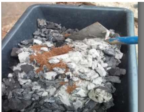
Figure 25 Dry mixing of different constituents of concrete
