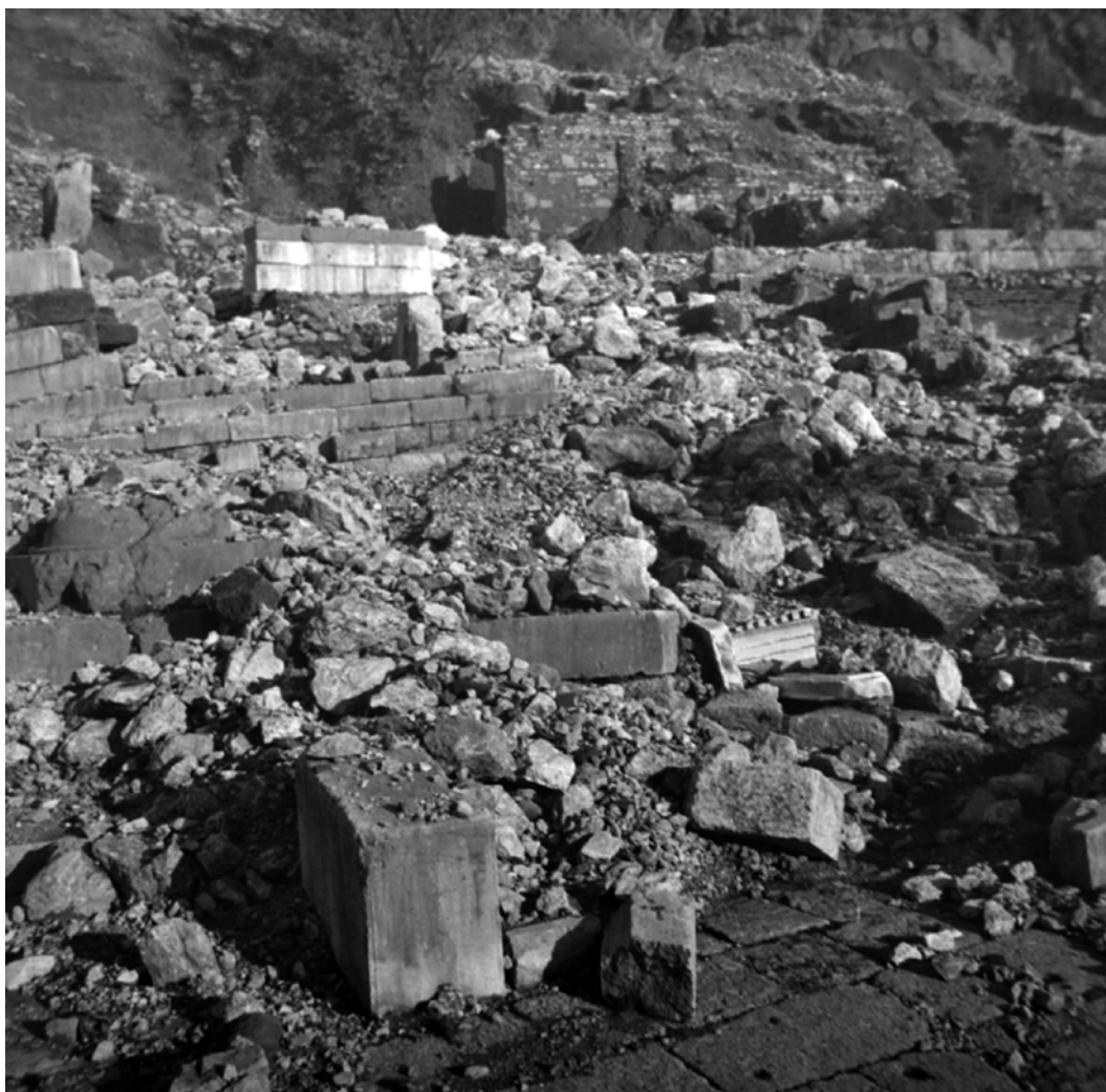
Figure 6: December, 1935. Deposits left by the catastrophic flood event over the Sanctuary of Apollo (French School at Athens).
