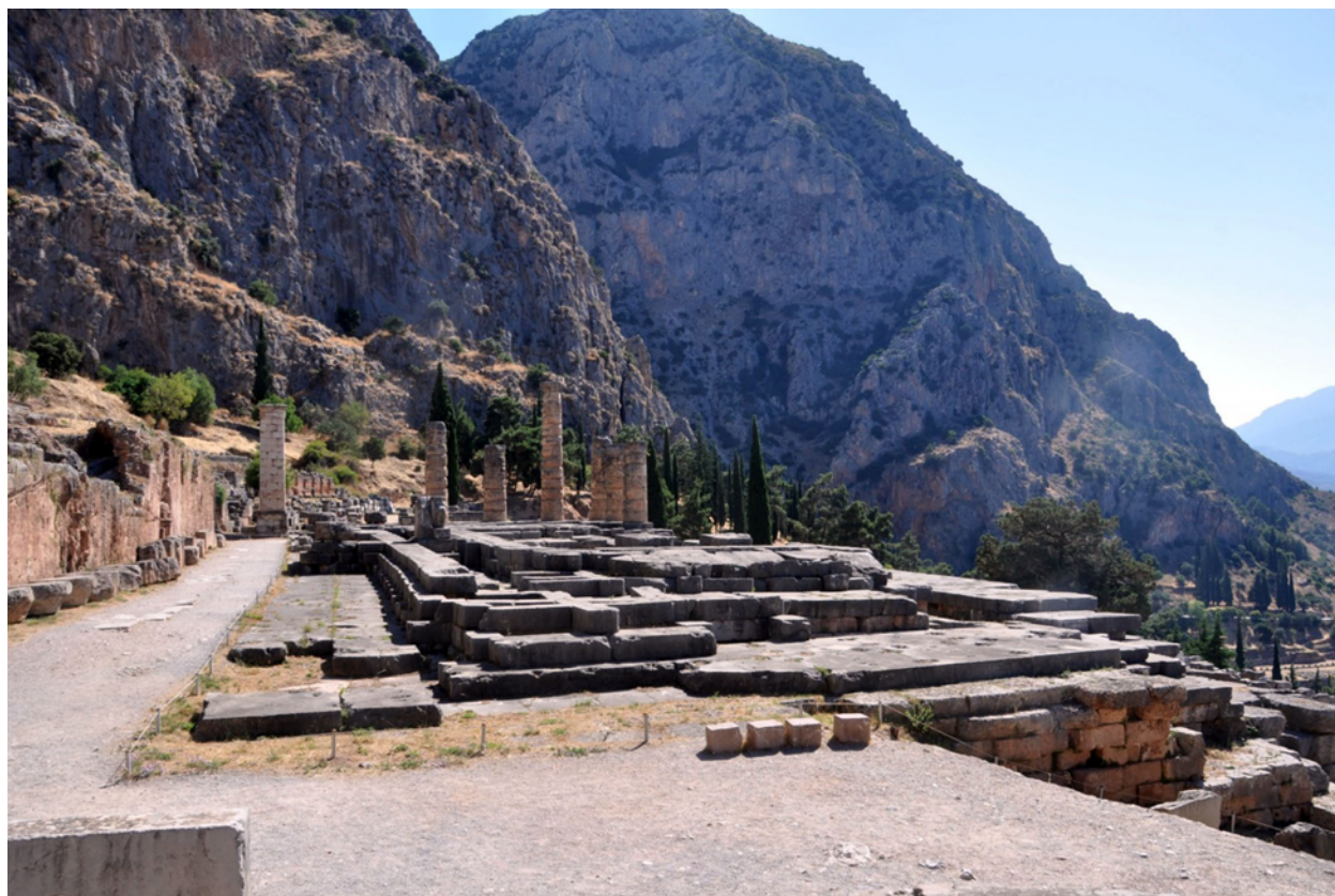
Figure 8: Temple of Apollo. Distortion of the euthynteria .
