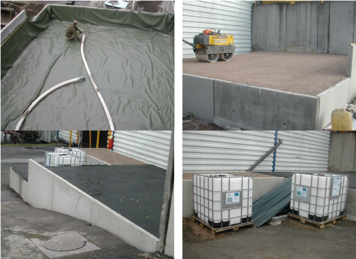
Figure 6 – Construction of the road structure for the test of lime-based binder (used in treated embankment).
