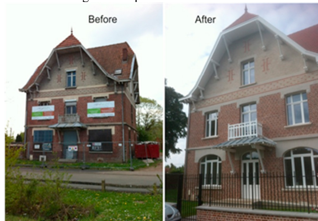
Fig. 1. Rehafutur: before and after renovation
