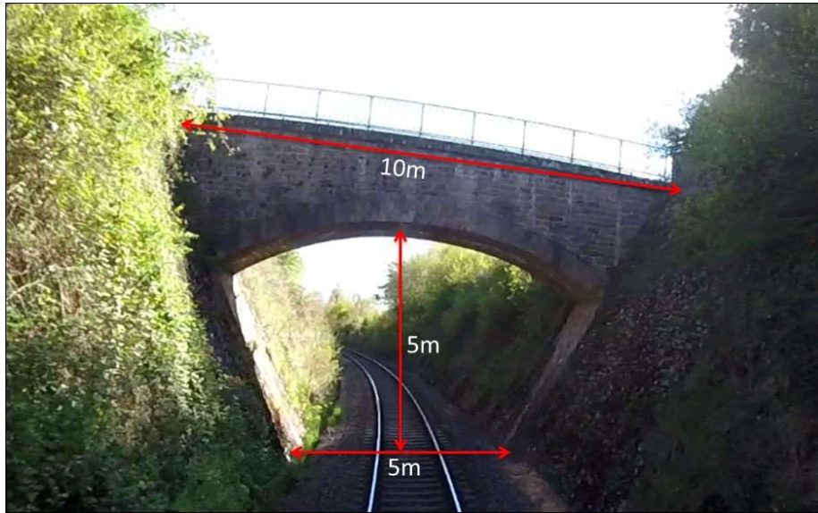
Figure 20: Railway bridge present on regional lines
