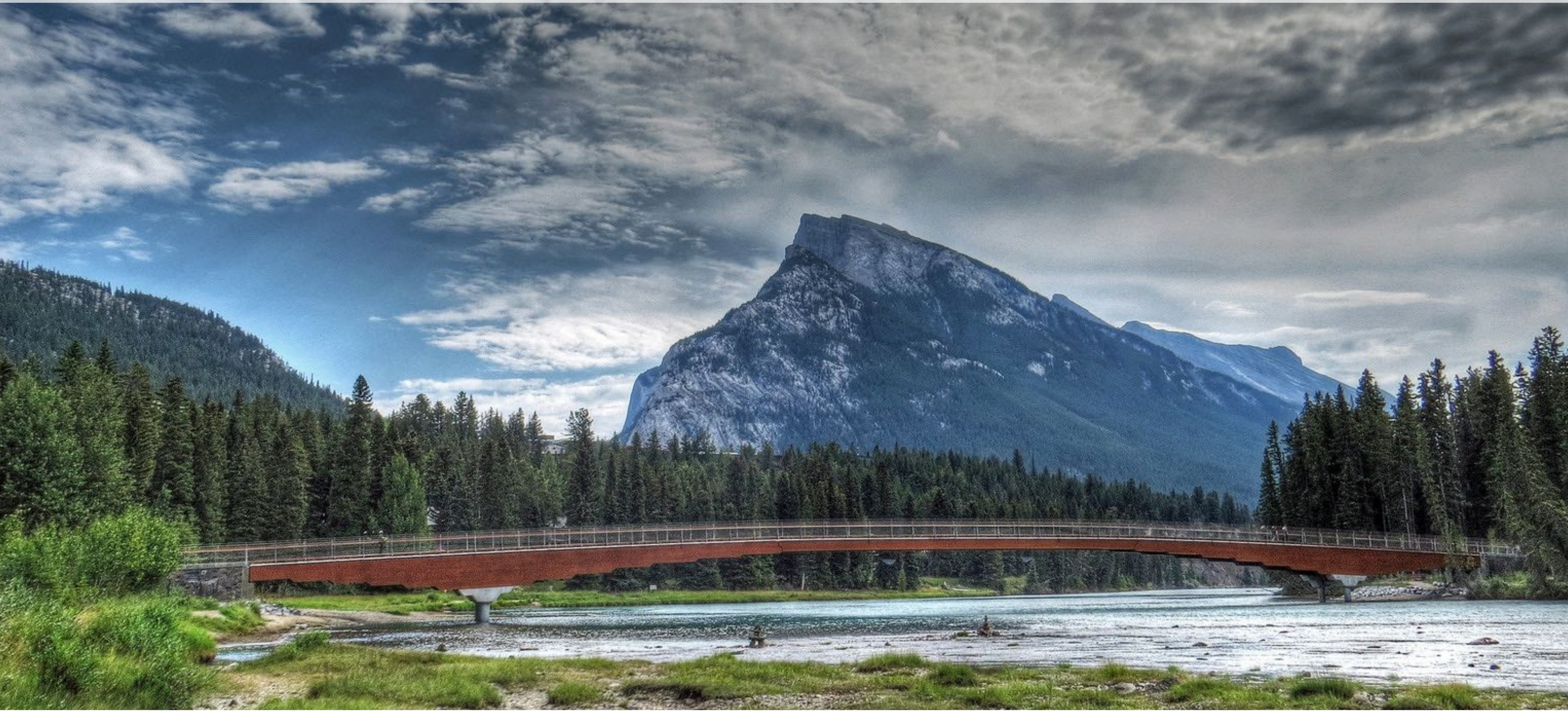
Bow River pedestrian Bridge (CA)
