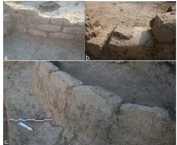
Figure 8: Plano-convex mud-bricks from Mentesh Tepe. a.: Detail of the four courses of mud-bricks, wall 293 (Sector 10) – View from the West; b.: Detail of the mortar between the mud-bricks, the wall 293 – View from the West; c.: Detail of the first course of mud-brick, wall 285 (Sector 15) – View from the North-East (Mission Mentesh Tepe).
