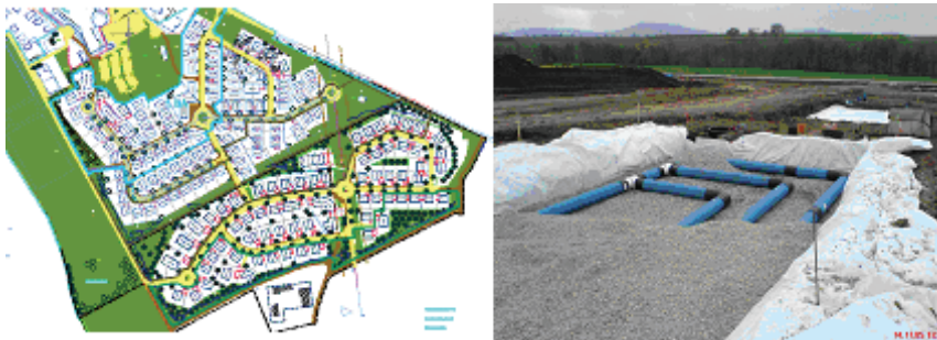
Figure 5 : Semi-central trough-trench-system in Kupferzell
