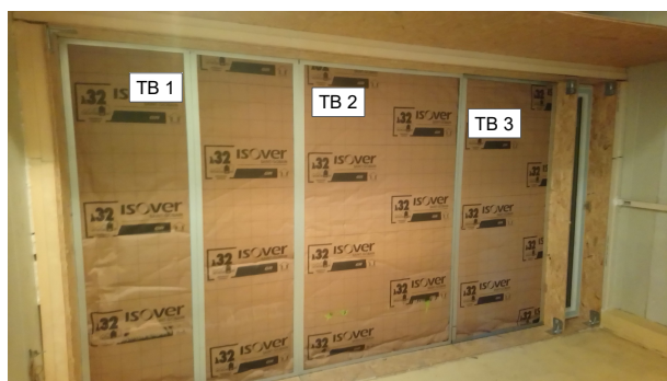
Figure 3: Photography of the wall before installation of the gypsum boards.
