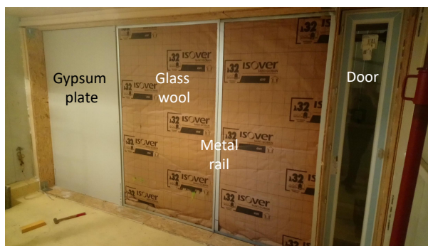
Figure 2: Photography of the wall before installation of the last gypsum boards.
