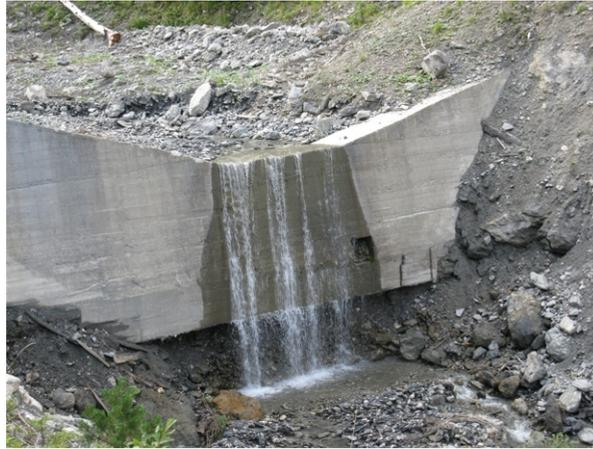
**Figure 3:** Scouring phenomenon downstream a check dam. Saint Antoine torrent, France, 2014. Source: ©INRAE/ETNA.
