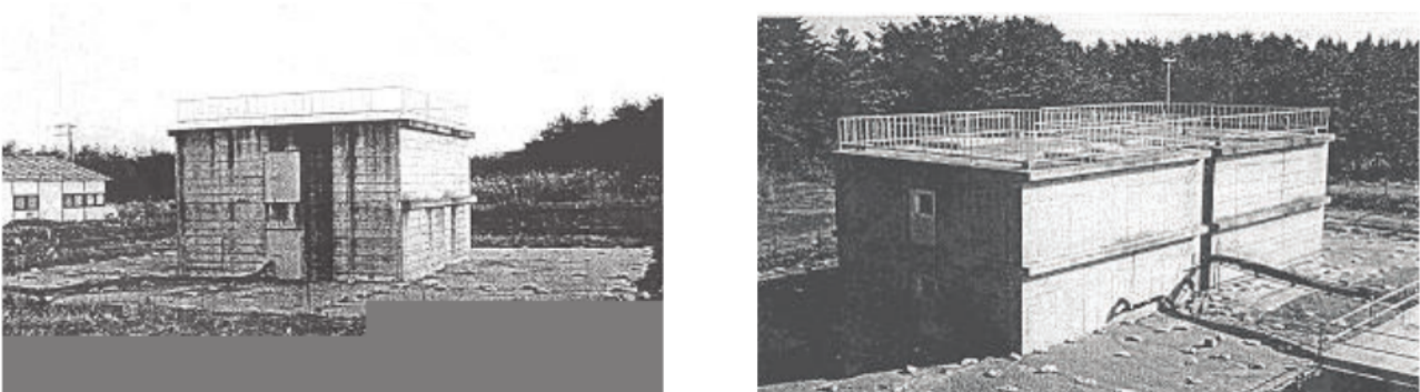
Figure 3: Single embedded building (top) and two identical closely spaced embedded buildings (low) [4]
