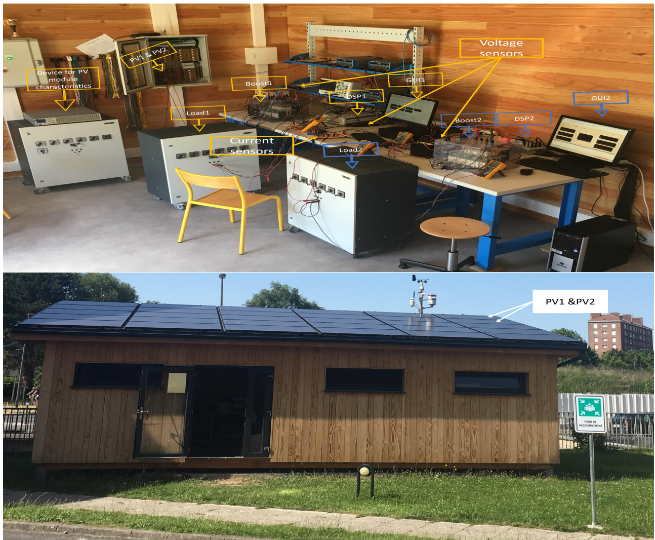
Figure 9: Different required devices used for practical experience.
