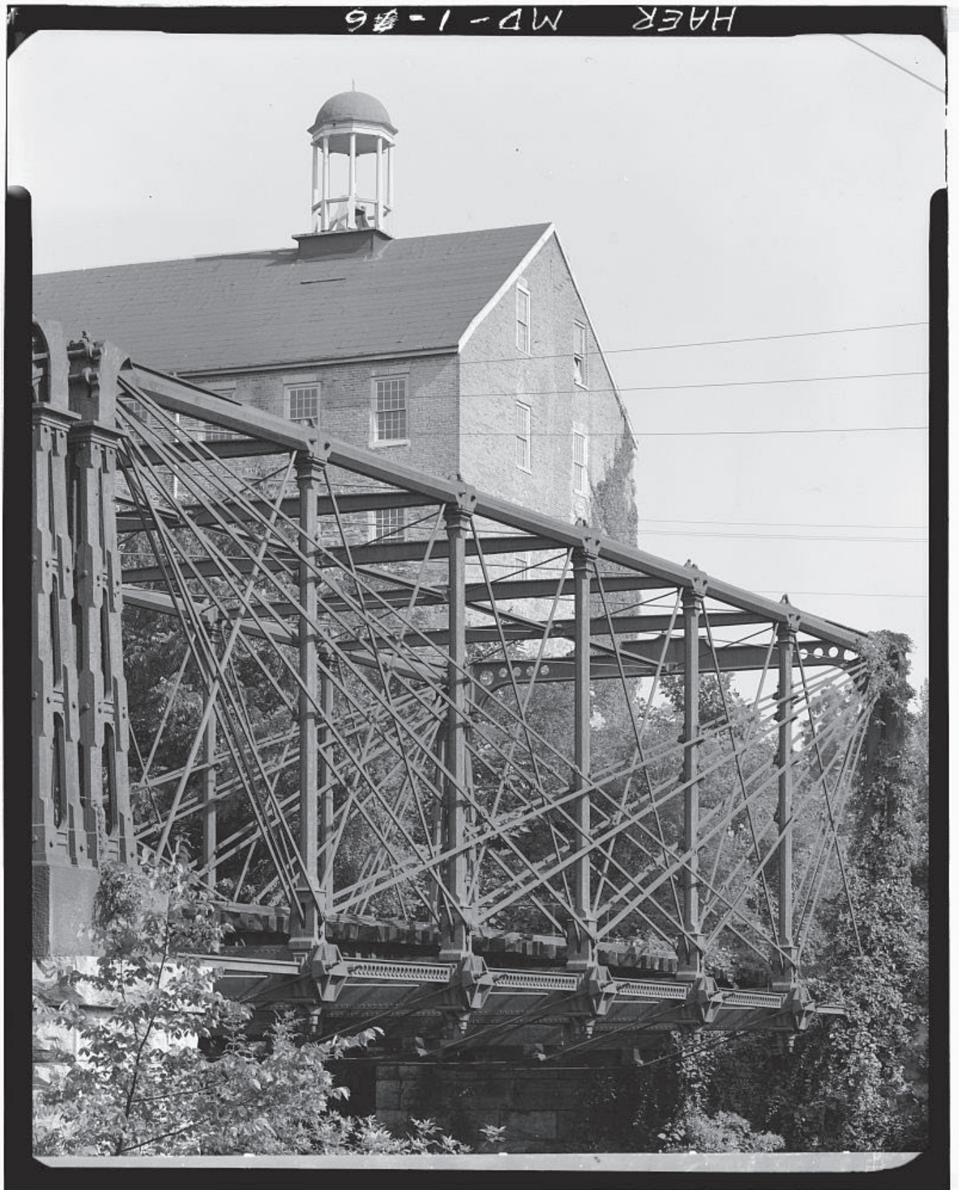
Bollman Truss Railroad Bridge, Savage mill, Howard County, MD Historic American Engineering Record - Library of Congress
