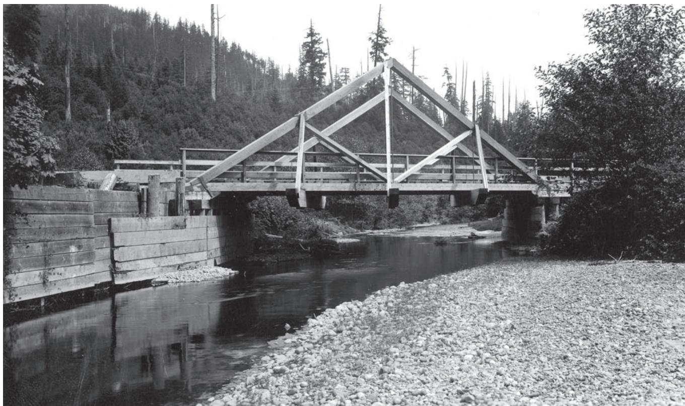
ci-dessus: l'archétype du pont primitif de type "King post", transposition d'une simple charpente Bandaret Bridge, Issaquah Creek - photo T.P. Blum 1933 source http://www.kingcounty.gov/depts/records-licensing/archives/exhibits/BlumBridges.aspx
