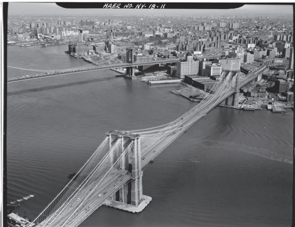
Brooklyn Bridge, Spanning East River, Brooklyn, New York, New York County, NY Historic American Buildings Survey/Historic American Engineering Record - Library of Congress
