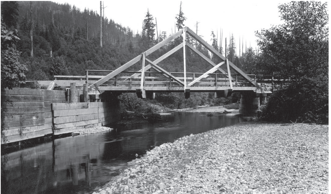
ci-dessus: l'archétype du pont primitif de type "King post", transposition d'une simple charpente Bandaret Bridge, Issaquah Creek - photo T.P. Blum 1933 source http://www.kingcounty.gov/depts/records-licensing/archives/exhibits/BlumBridges.aspx
