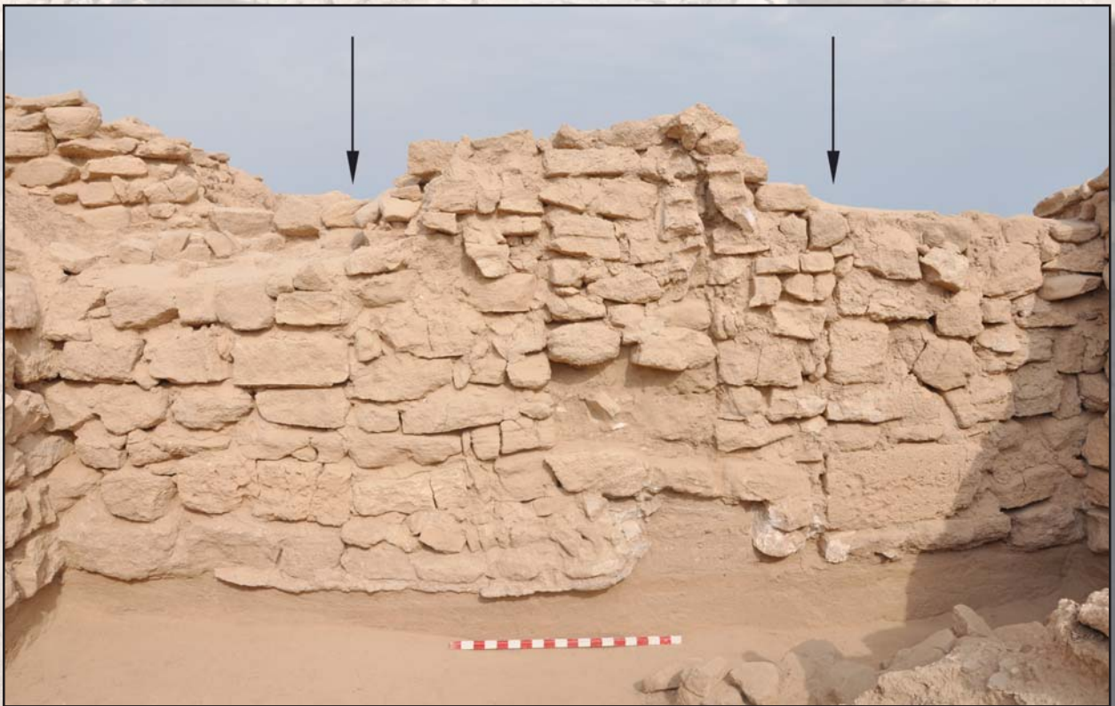
B sector , tower 6. The north door and the two fill-in ; the arrows show the first entrance. View to the north.
