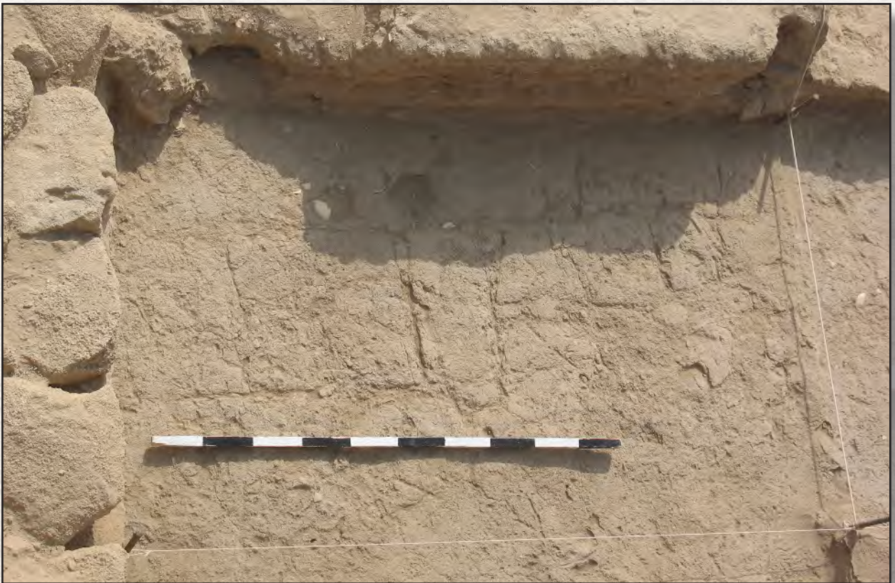
C3 sector. Detail of the mud brick wall M365.
