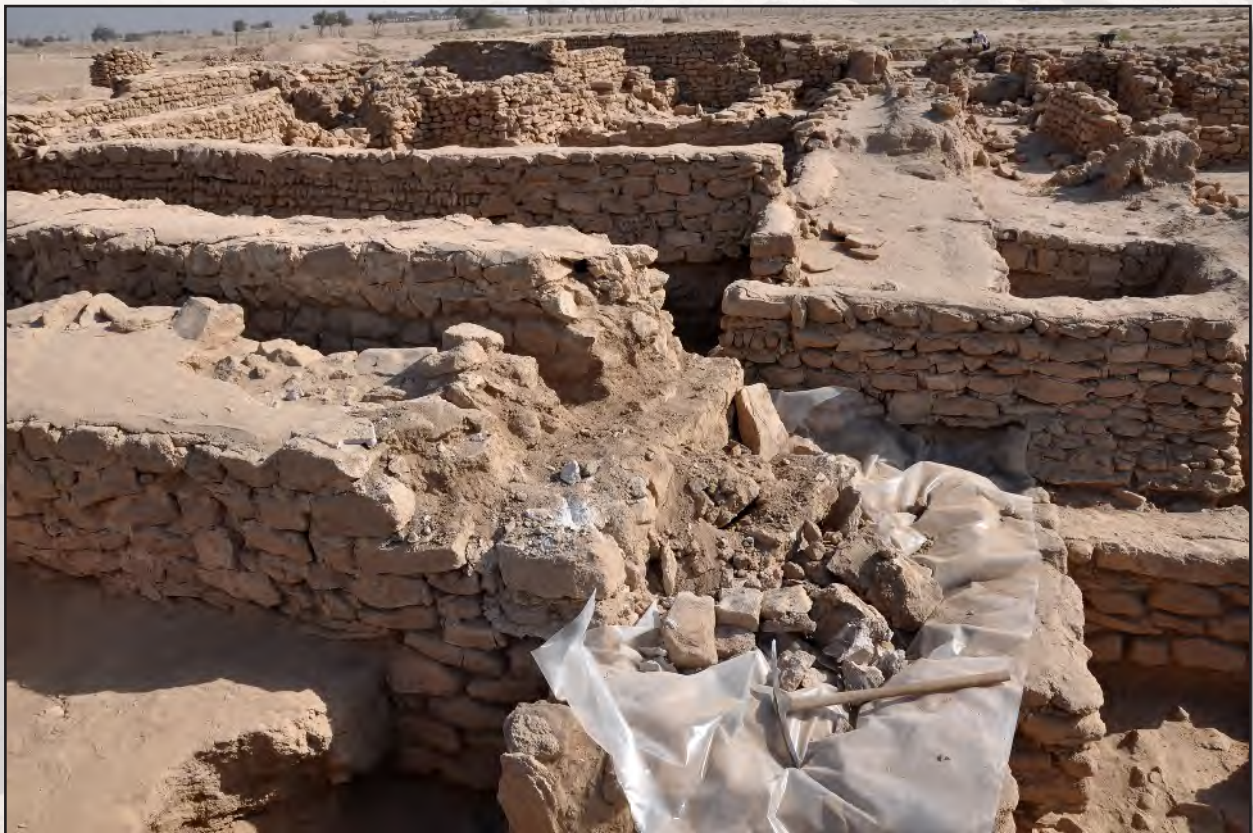
A2. Removal of the cemented wall which was linking the tower 2 (on the left) and the latest corridor wall M301, to reconstitute the state after ancient excavations. The cemented wall M348C, just after the nylon, has been removed too. View to the east.
