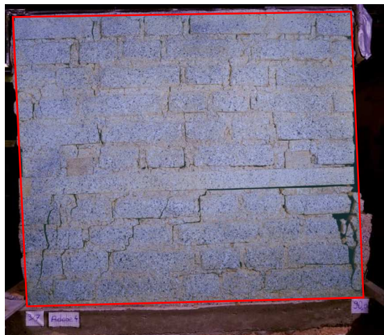
Fig. 14 Wall with timber band at 4560 seconds of loading at peak displacement towards left
