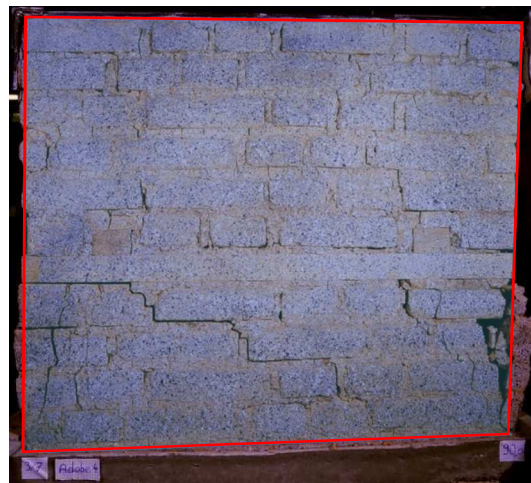
Fig. 15 Wall with timber band at 4880 seconds of loading at peak displacement towards the right
