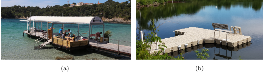
Figure 2: (a) Pontoon of Pierre Caron (France). (b) Modular floating dock system Candock®.
