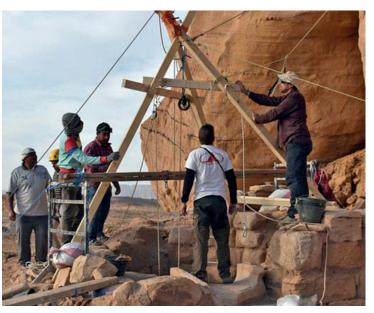
**Fig. 23.** Well no. 132, the two rock climbers finishing the installation of the lifting jack.
