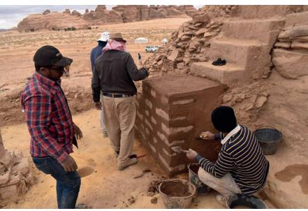
**Fig. 30.** Building of the staircase to secure access to the top of IGN 132.
