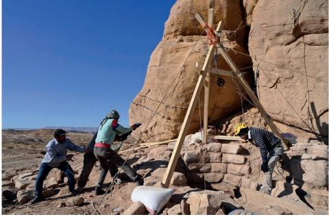
Fig. 4. The lifting jack installed over well 132 in order to empty it.
