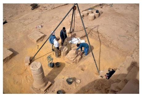
**Fig. 27.** The two columns in situ before the beginning of the restoration and the lifting jack.
