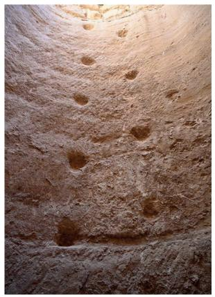
Fig. 24. Notches cut in the wall of the well.
