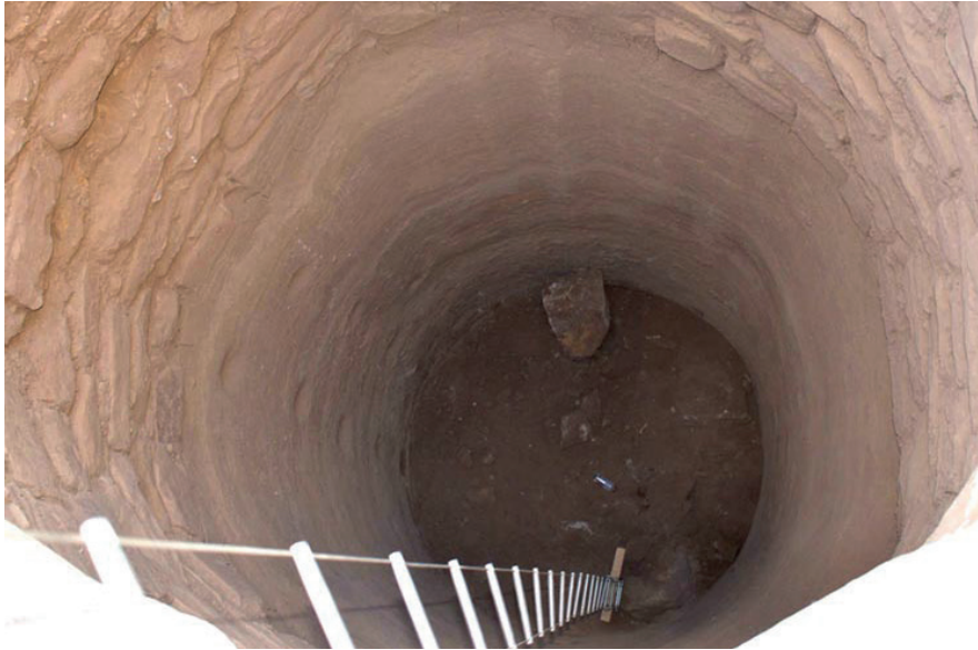
Fig. 26. View of the inside of the well.
