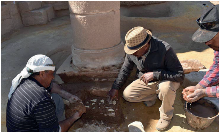
Fig. 31. Consolidation of the base of column 66022.
