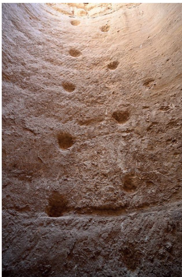
Fig. 6. Notches cut in staggered rows in the well.
