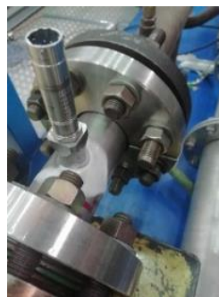
Figure 2. Piping demonstrator with its pressure/temperature probe mounted in the aeraulic test bench.
