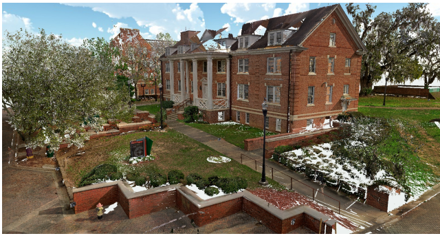
Figure 6: 3D point cloud data from laser scanning done on FAMU campus.
