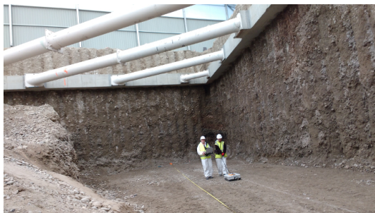
(a) GPR acquisition along a longitudinal profile.
