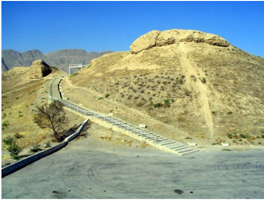
Stairs bringing visitors from the parking area to the top of the ramparts
