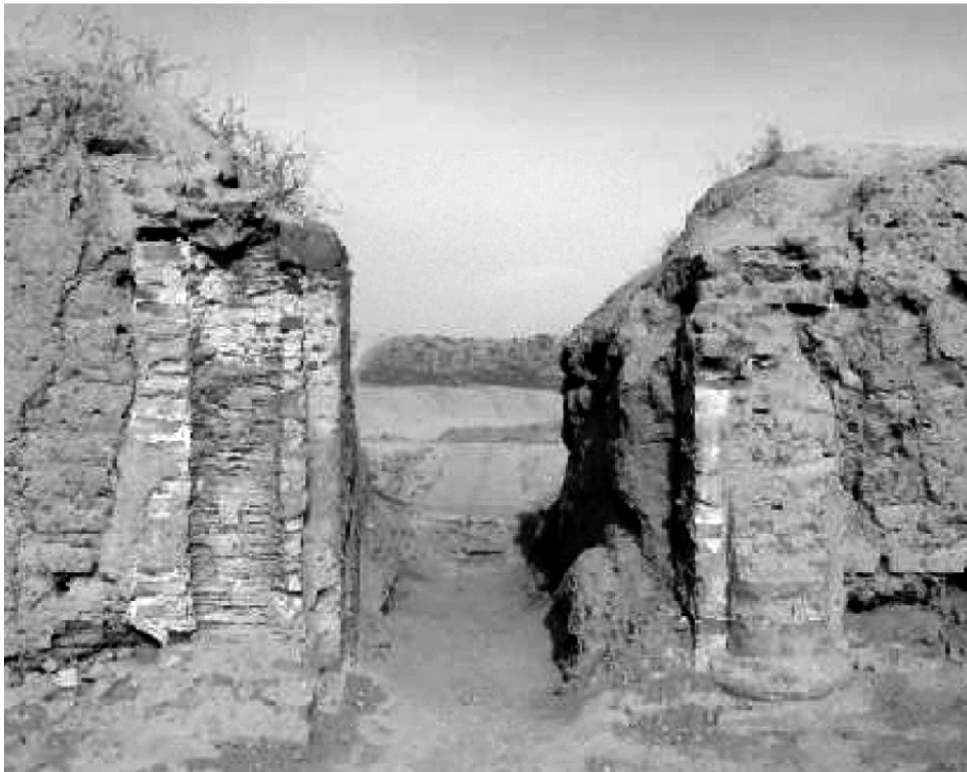
The columned hall
