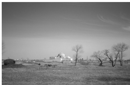
Empty land surrounding section 3
