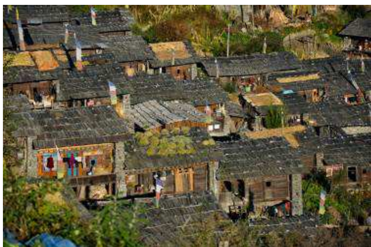
Fig.8) Row houses in Gatlang before Gorkha EQ
