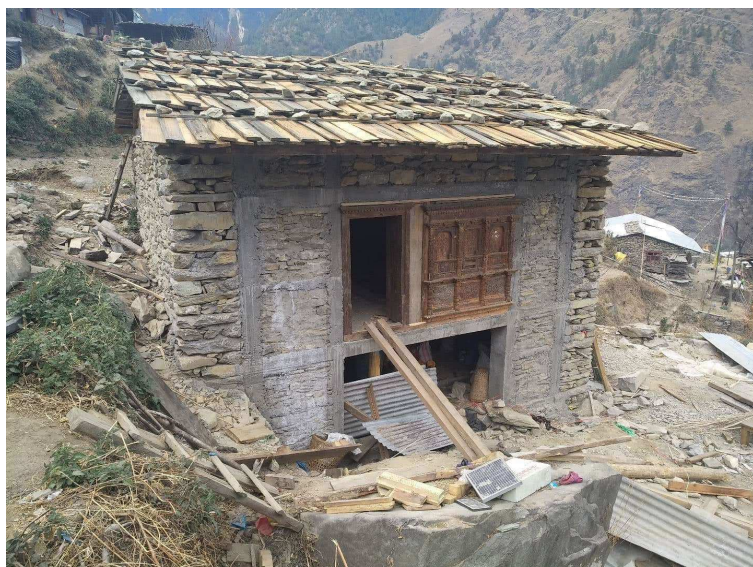
Fig. 31) Gatlang, retrofitted house using “strong back” approach 16
