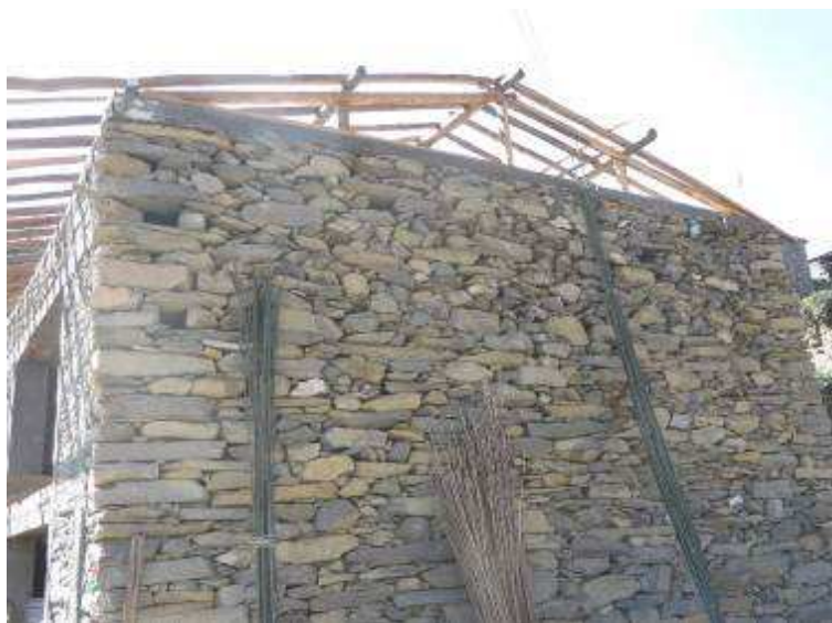
Fig. 32) Gatlang, retrofitted house using “strong back” approach 17
