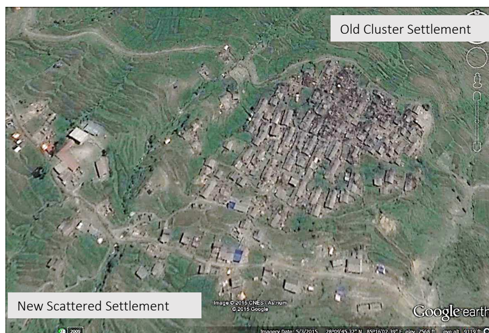
Fig.6) Top view of the village of Gatlang after 2015 EQ. (Source ASF Nepal report)
