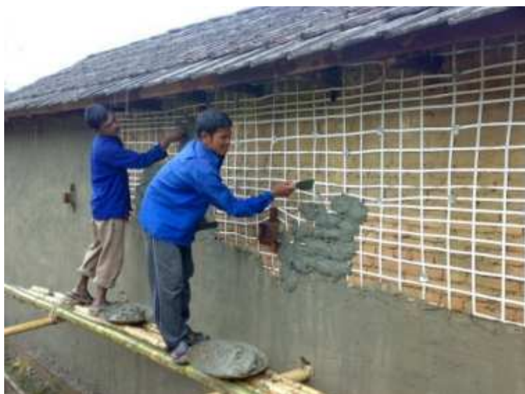
Fig. 37) NSET, Implementation of PP band method of retrofitting in Kathmandu Valley 21
