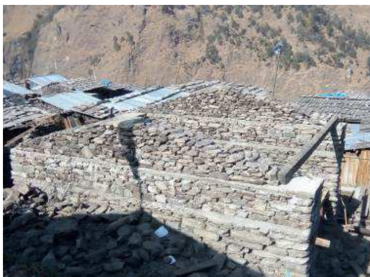
Fig. 33) Repairs and reconstruction of gable wall (confined) in Gatlang, ASF Nepal /CRAterre 2017
