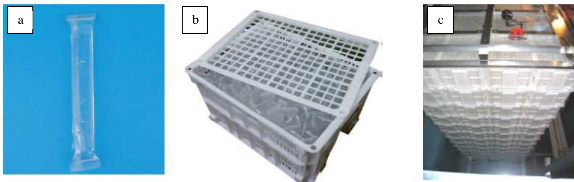
Figure 3 – (a) Latent Heat Thermal Storage material package (gel pack), (b) plastic case filled with gel packs and (c) typical installation of the plastic cases into the isolated tank.
