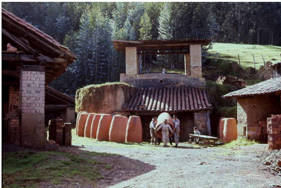
Figure 3. Carrying the moyas to the furnace at a salt works in Nemocón. 1970.
