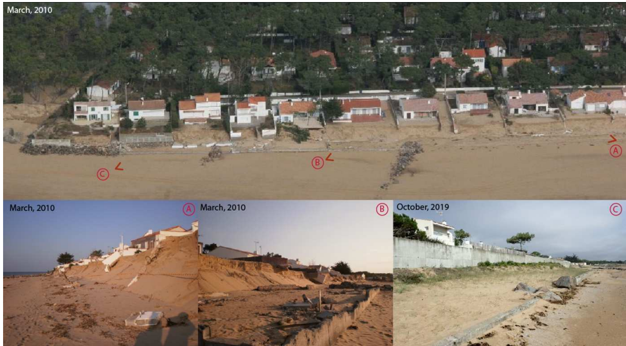
Fig. 4: The shoreline’s retreat and damage on protection works in the aftermaths of Xynthia. La Tranche-sur-Mer – South of the Clémenceau beach
