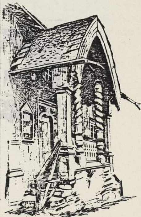
ASSISE HOUSE AT SUNDE AALL, HALLINGDAL, BUILT BY JOLLEF VILLAND DRAWN BY WILLIAM PETERS
