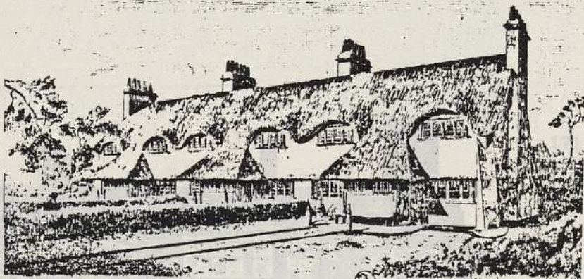
SIX COTTAGES AT ELMESTHORPE NEAR LEICESTER FOR THE EARL OF LOVELACE. C.F.A. VOYSEY, ARCHITECT
