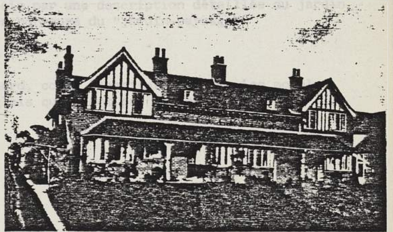
BOURNVILLE: COTTAGES IN LINDEN ROAD (BACK VIEW)
