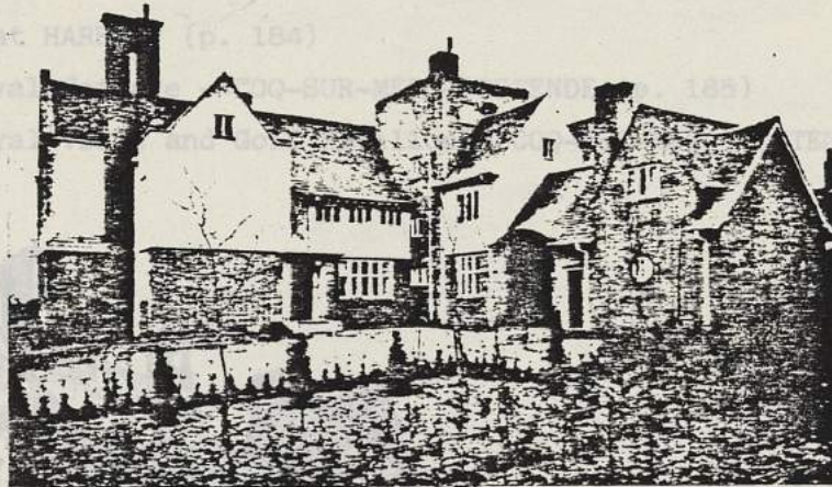
"GARTH HOUSE," EMBAYSTON: DRIVE FRONT
