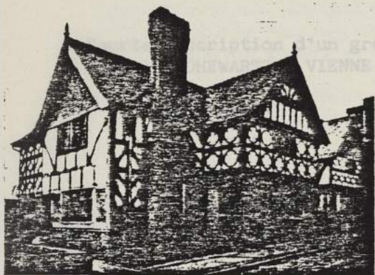
COTTAGES IN MANOR ROAD, THORNTON HOUGH
