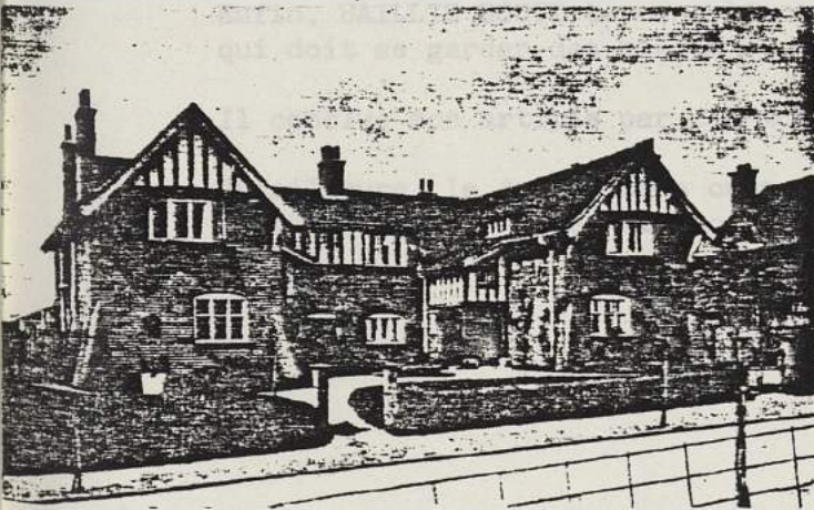
BOURNVILLE: COTTAGES IN LINDEN ROAD (FRONT VIEW)
